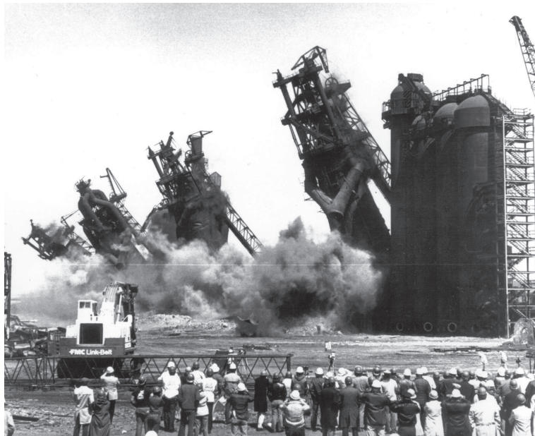
The implosion of US Steel's Ohio Works.
